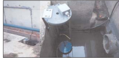
Figure 5. Rain water run off from bunded area
